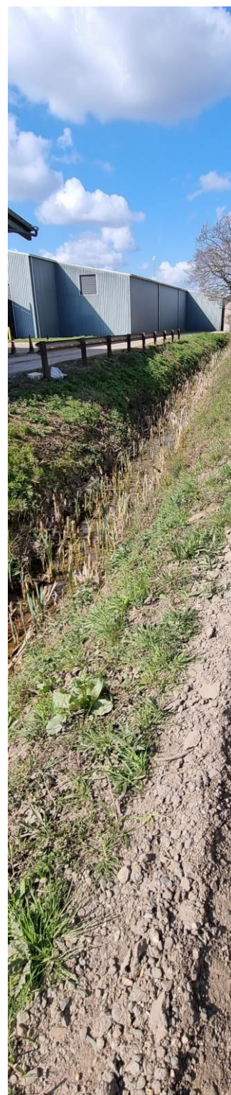
Fig. 10.1 Reedbeds established naturally in the base of a larger ditch – the water teeming with pondlife.
